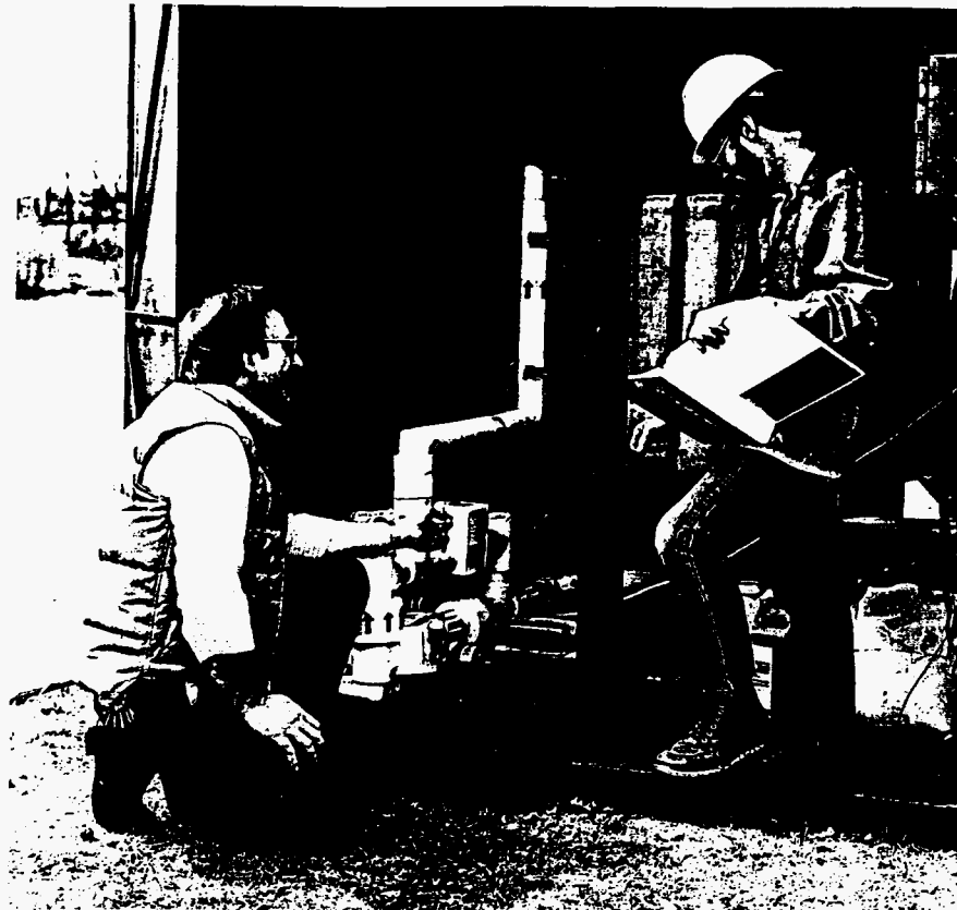
On-site staff adjust nutrient storage and delivery equipment to maintain appropriate injection of nutrients.
