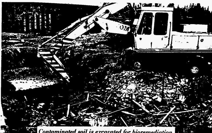
Contaminated soil is excavated for bioremediation
