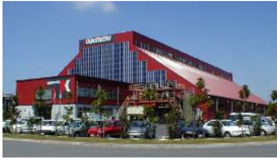
Figure 58 : Installation Thermoselect de Chiba (Japon)
