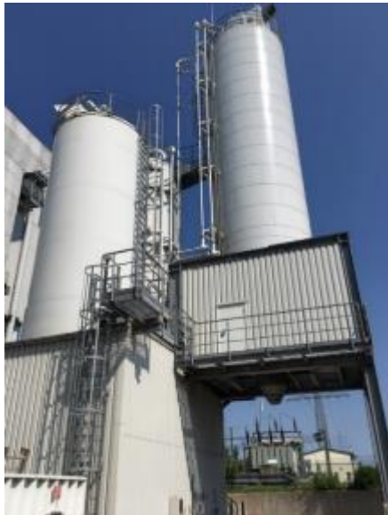
Figure 80: Silo cendres volantes (RECORD, 2018)
