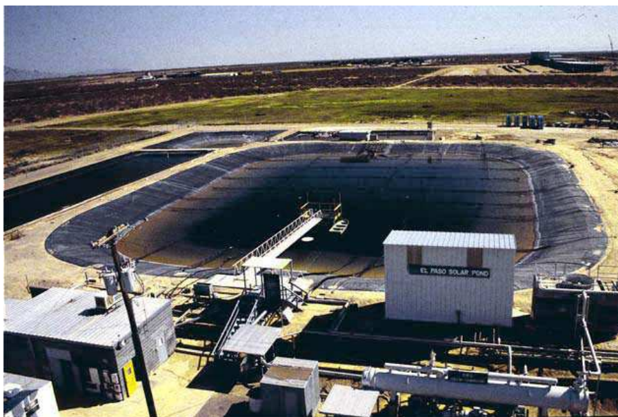
Figure 4.2 : Etang solaire de El paso (University of Texas USA)
